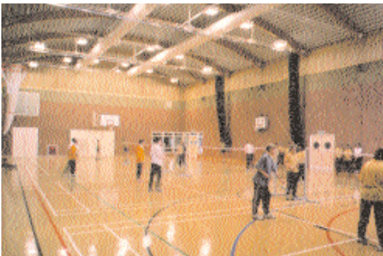
A successful sports hall interior with walls of masonry block and a slatted timber band for sound control. All these materials have around 50% reflectance value.
