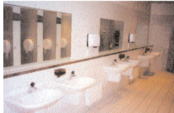
Basin ducts protect pipework and simplify surface cleaning. In this example 'between basin' dispensers help conceal any soap spillage.
