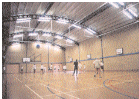
Radius'd steel cellular beams and a structural ceiling liner give this sports hall an uncluttered appearance.
