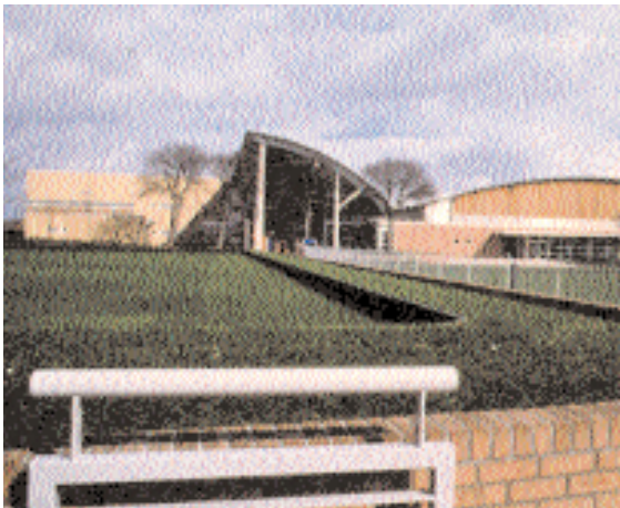
The sports centre in its setting: interesting building forms invite attention.
