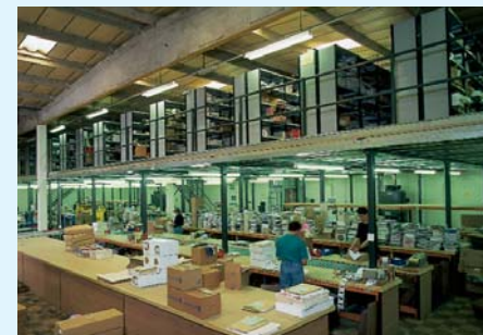
Mezzanines, two tiers and floorovers
