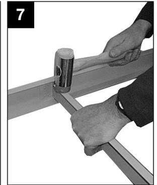
7. Locate Decking Supports. Slots in the decking supports locate into lugs at the centre of the beams.
